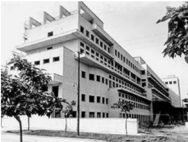
Figure 2.51. Original form of the Children’s Hospital on Tiršova Street. Photo credit: Milan Zloković (via the Milan Zloković Foundation).
