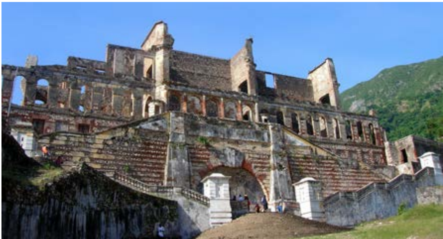
Figure 2.138. Recent photo of the Sans-Souci Palace, showing the symmetrical stairs. Photo credit: Rémi Kaupp (via Wikimedia Commons), CC BY-SA 3.0.
