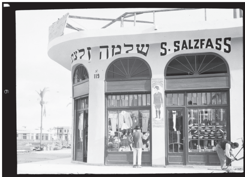
Fig. 2: "Man looking at the display window of a menswear shop," NINO, F. Scholten, Jaffa-Tel Aviv-Sarona , 09:020. The shop's façade looks like it has been renovated only recently, adding to the new appearance of Tel Aviv's center. A first window shopper inspects the new wares.
