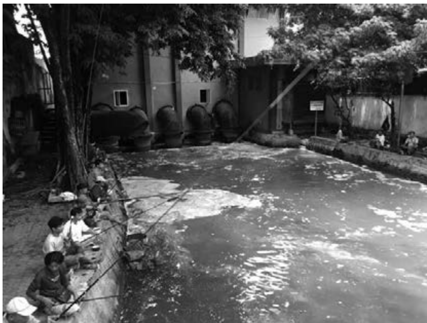
Figure 2.4 Massive pumps discharge excess water from low-lying districts into the Kali Mas, providing a good spot for Sunday morning fishing (Photo by Howard Dick, December 2017)
