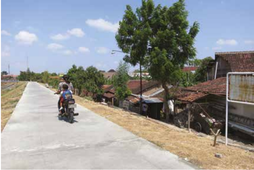
Figures 7.9 and 7.10 Embankments along the Bengawan Solo River and gabion walls along the Code River provide protection from flood (Photos by the Author, 2012)
