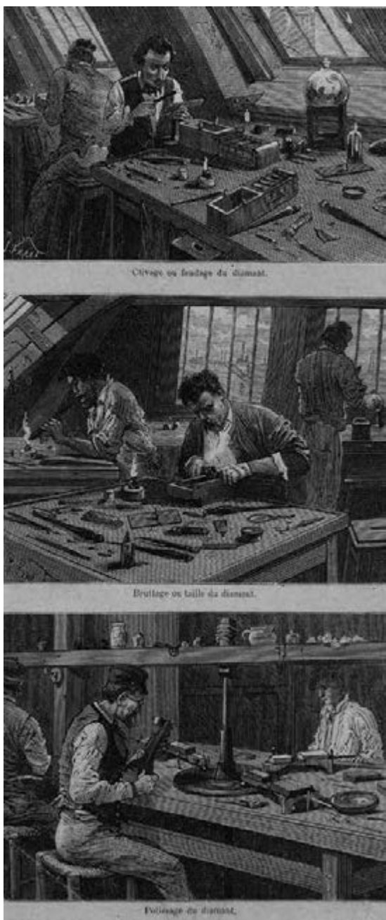
Figure 4.5 The main operations of diamond processing: splitting, cutting, polishing, c. 1880
