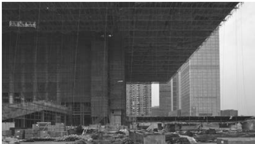
Figure 10.8. Worksite at Shenzhen Stock Exchange. Video still from Zachary Formwalt, Unsupported Transit , 2011.
