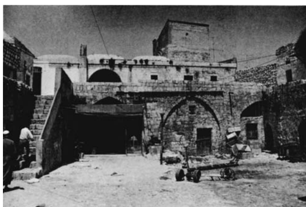
Plate 47.4 North end of courtyard
