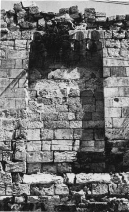
Plate 54.4 Blocked window at west end of upper floor façade
