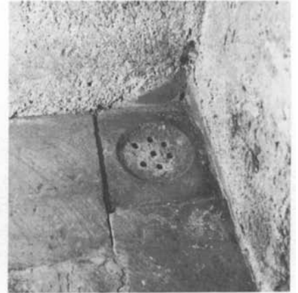
Plate 36.24 Upper floor: drain in floor of bath-house
