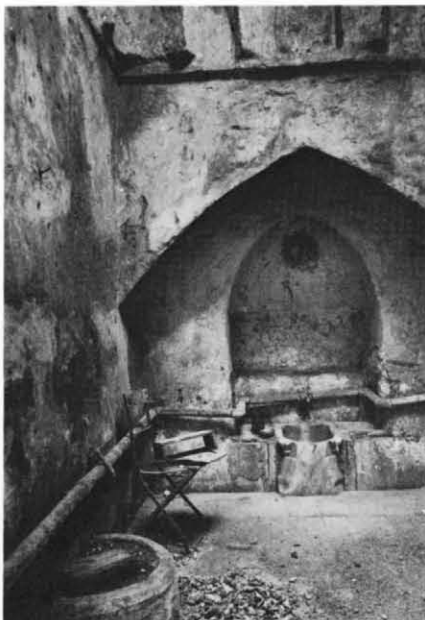
Plate 24.33 Hammām al-'Ayn: eastern subsidiary hot room – recess in south wall
