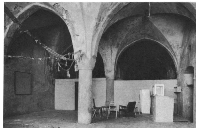
Plate 5.6 Main hall, looking south
