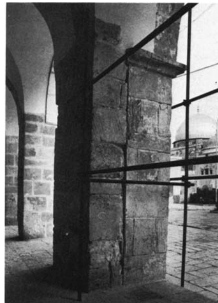
Plate 12.1 Pier 54: south-east corner
