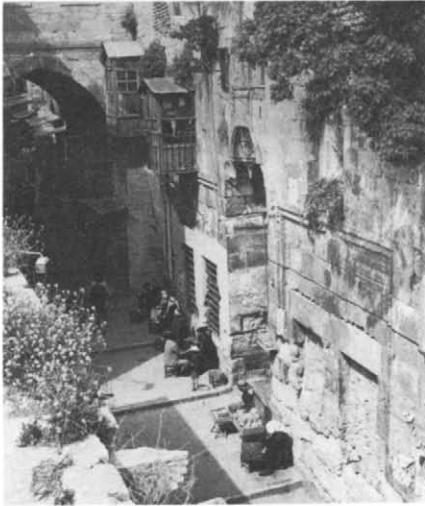
Plate 29.1 Street façade from south-east
