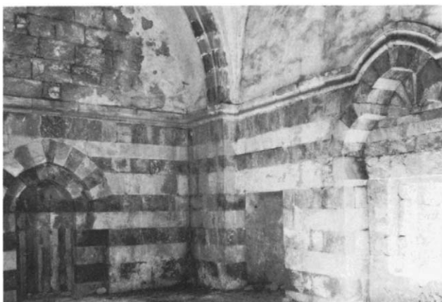
Plate 31.11 Assembly hall, south-west corner
