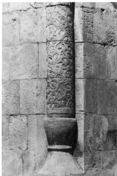
Plate 64.5b South-east corner shaft
