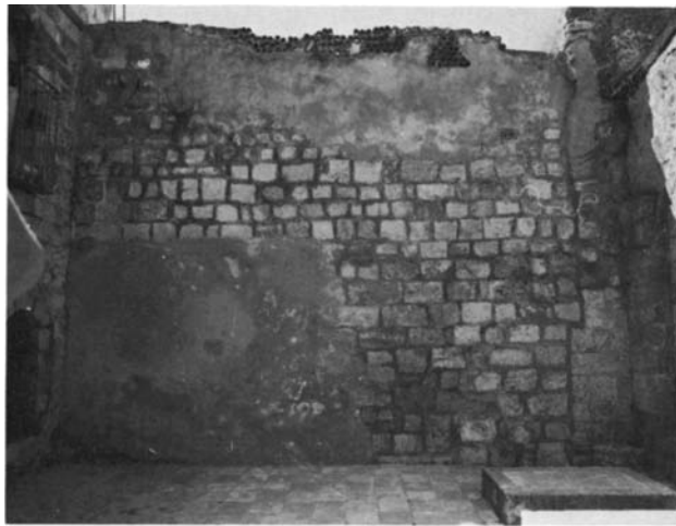
Plate 2.9 South side of courtyard
