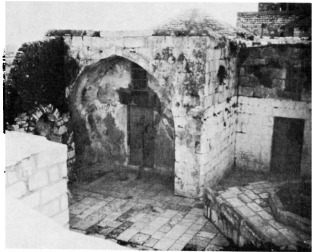
Plate 45.16 Roof court: south-east corner
