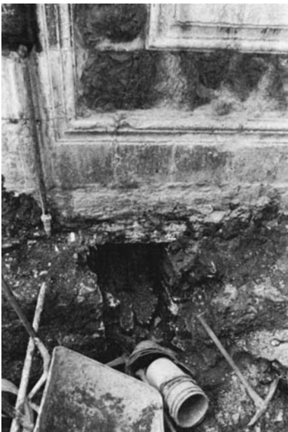
Plate 48.25 Drain under eastern portal
