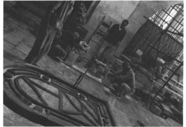
Plate 17 Qamariyya mould prepared to receive plaster
