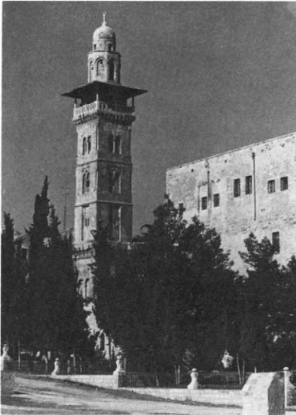
Plate 10.1 General view from the south-east
