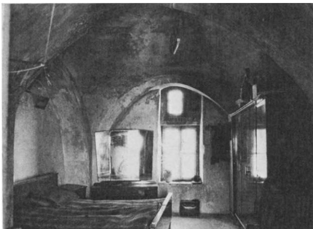
Plate 25.7 Upper floor room with window to balcony
