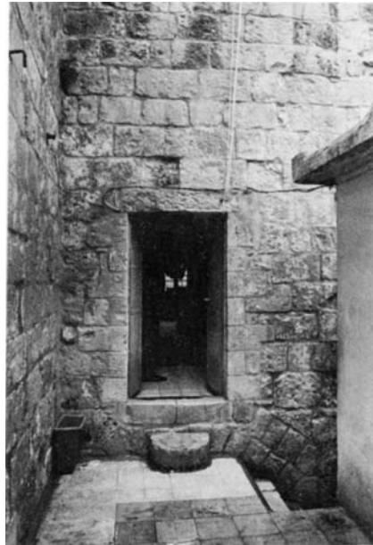
Plate 43.20 Modern entrance to south-west mezzanine
