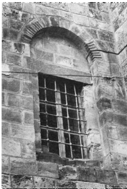
Plate 55.3 Window showing original grille
