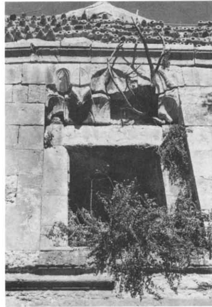
Plate 29.4 Upper-level window of eastern tomb chamber
