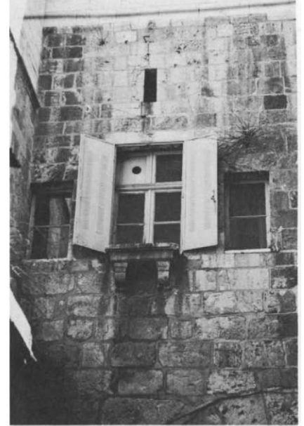
Plate 35.23 Windows in west wall of hall 'M'
