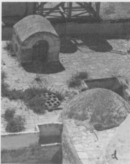
Plate 18.23 Roof of rooms 'O', 'P' and 'L'
