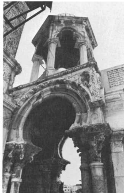
Plate 27.3 Domed pavilion and horseshoe arches from the east
