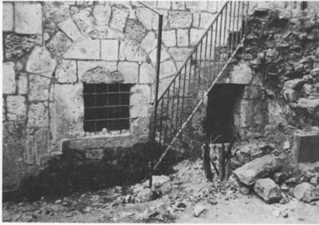
Plate 34.1 Street frontage after removal of stair to upper floor
