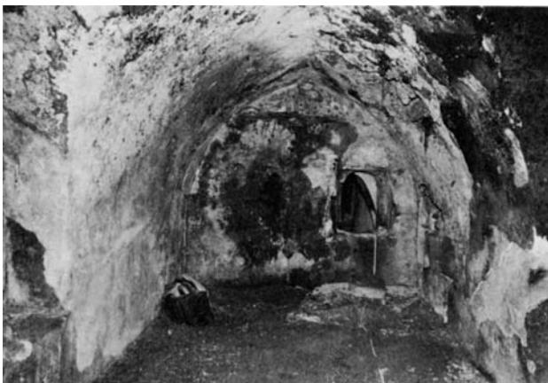
Plate 43.22 North-east mezzanine looking south
