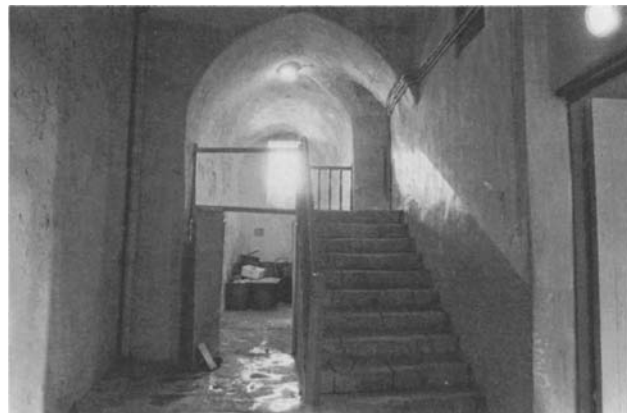
Plate 18.10 Staircase from entrance vestibule to upper floors
