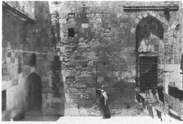
Plate 25.9 South end of west wall of courtyard
