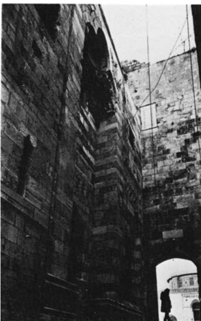
Plate 61.1 Street façade from south-west
