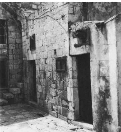
Plate 36.15 Upper floor: south-west corner of courtyard
