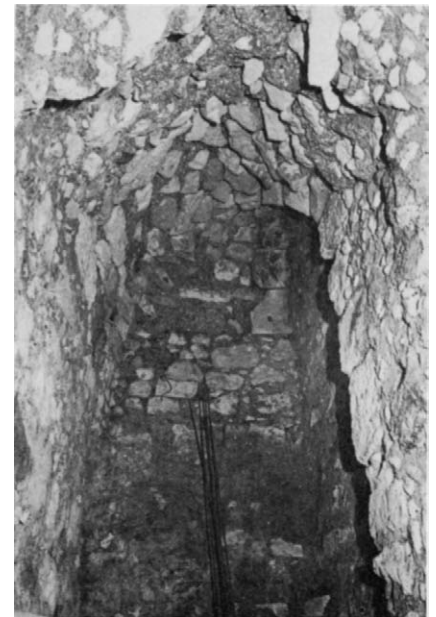
Plate 40.13 Rising vault at north end of passage
