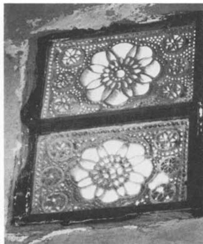
Plate 31.9 High-level window to courtyard from assembly hall
