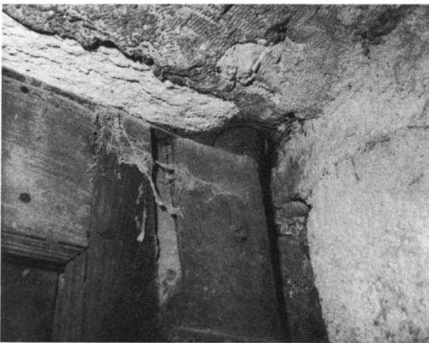
Plate 12 Hinge pivot in socket in lintel of entrance to Tashtamuriyya
