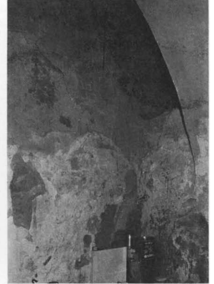
Plate 15.3 Rising vault over former staircase
