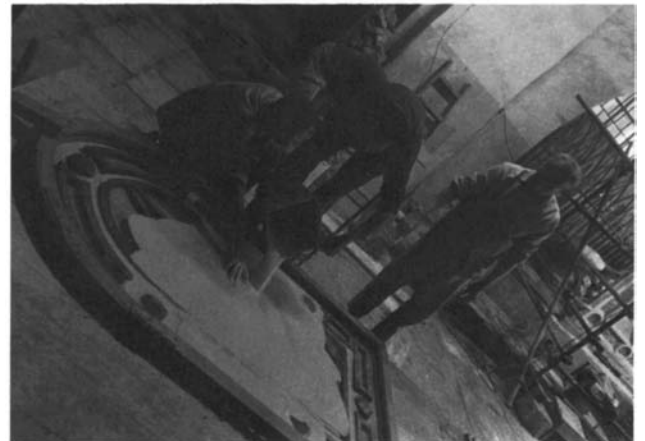
Plate 18 Pouring the plaster
