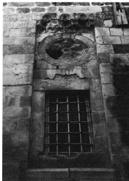
Plate 58.3 Right-hand window in upper storey façade
