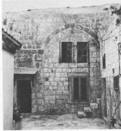
Plate 36.11 Upper floor: blocked iwān at south side of courtyard
