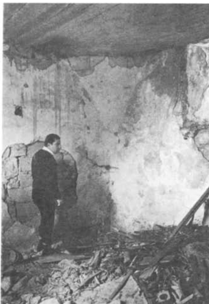
Plate 29.11 Pendentive in north-west corner of eastern tomb chamber
