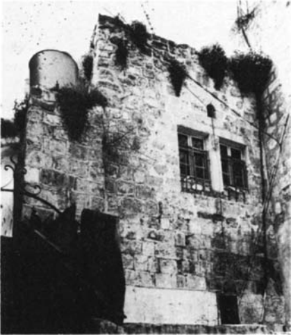
Plate 9.13 Upper part of south side of western courtyard
