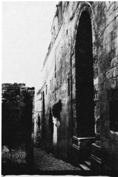
Plate 48.5 Street façade from west
