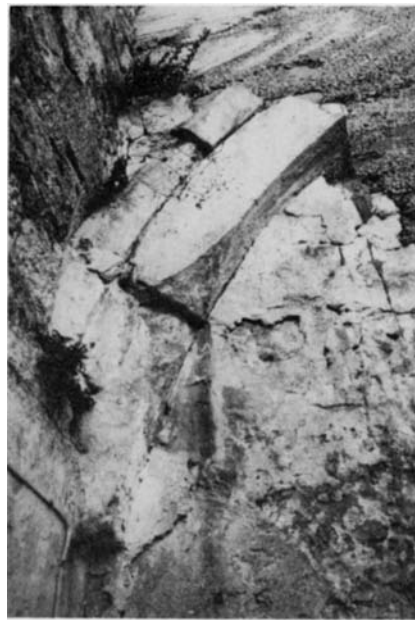
Plate 40.16 Upper floor: remains of arch at east end of south wall
