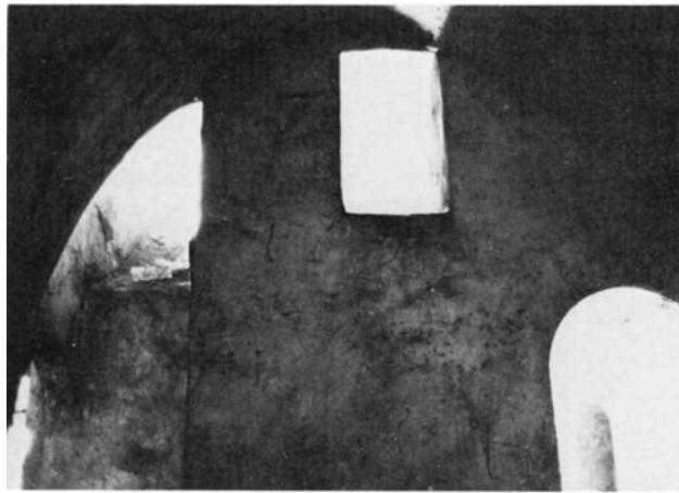
Plate 54.7 High-level windows lighting passageway
