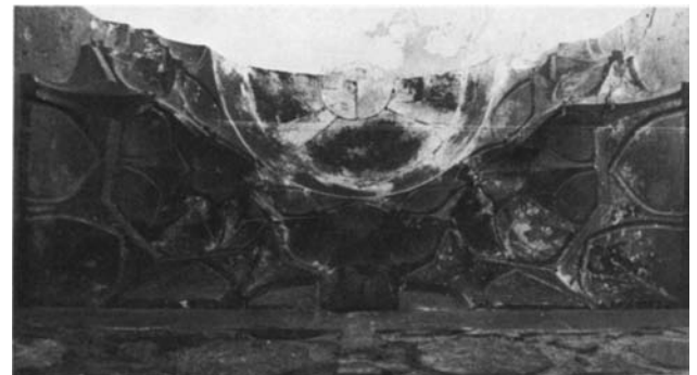
Plate 13.2 Vault of entrance portal from below
