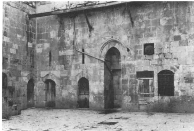
Plate 25.10 South end of courtyard with well-recess in centre
