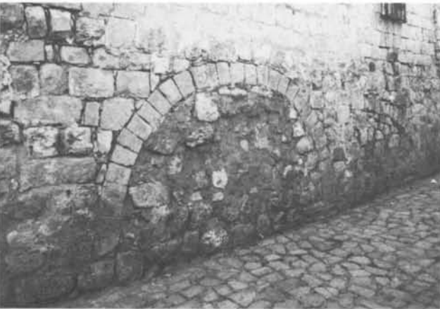
Plate 39.2 Arch in street façade
