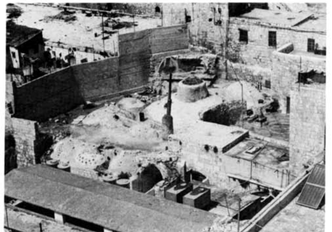
Plate 24.19 Hammām al-Shifā': general view of roofs from south-east
