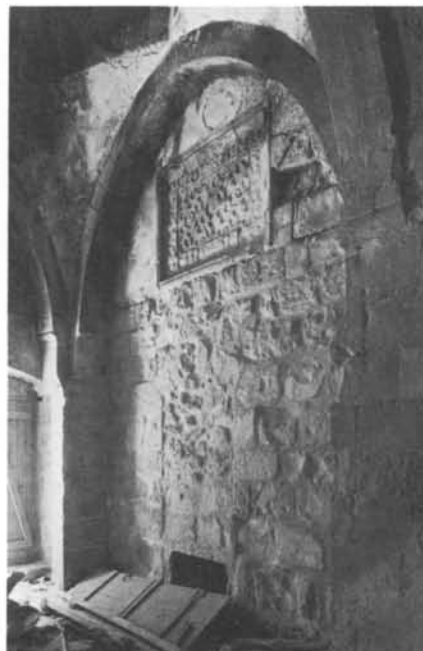
Plate 28.6 West wall of domed chamber
