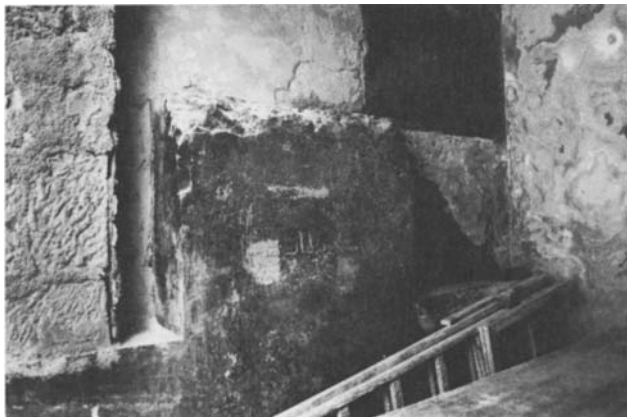
Plate 33.18 'Pilastered' masonry in south wall of tomb recess
