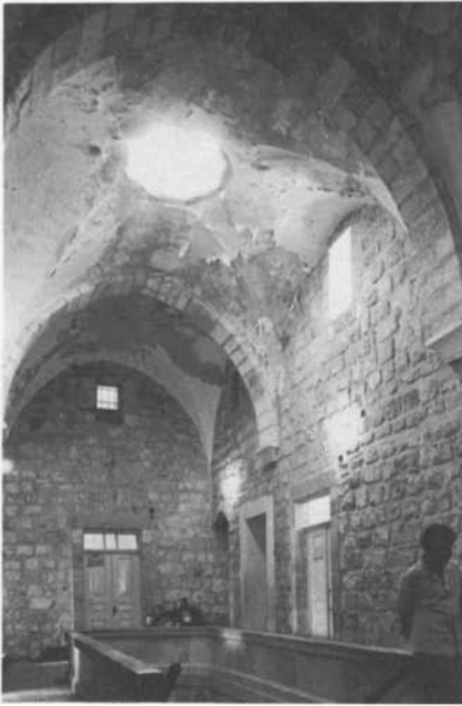
Plate 35.15 Gallery: looking south-west
