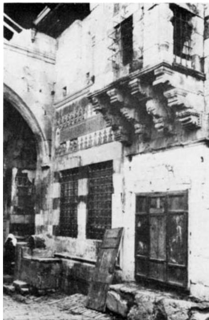
Plate 45.2 Façade (eastern half) with commercial unit of 3 shops and independent lodgings, rab' , above
