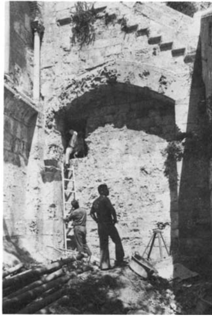
Plate 10.6 Arch supporting entrance stairs, under which an opening gives access to an old cistern
