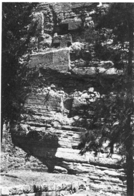
Plate 3 Antonia rock scarp showing beam socket (at top of plate) and remains of vaulting springer (below)
