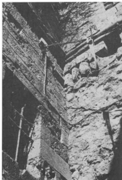
Plate 40.6 Moulding returning across street at north end of façade
