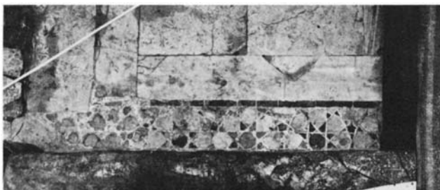
Plate 24.30 Hammām al-'Ayn: traces of polychrome marble pavement
