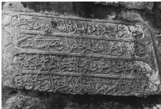
Plate 48.26 Upper floor: Ottoman inscription re-used in south side of courtyard
