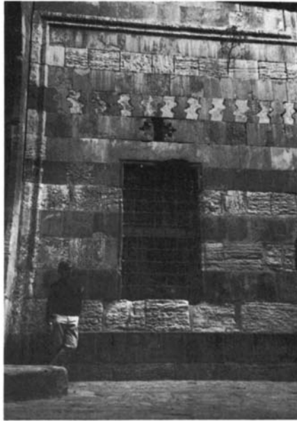
Plate 11 East end of Arghūniyya façade: note missing joggled inlay above window lintel
