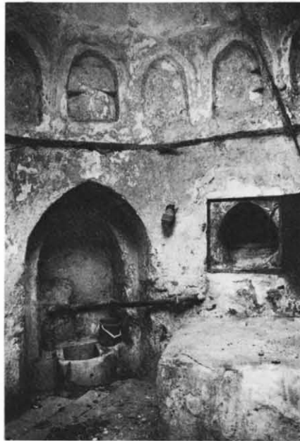
Plate 24.32 Hammām al-'Ayn: principal hot room – south-east recess (left) and boiler (right)
