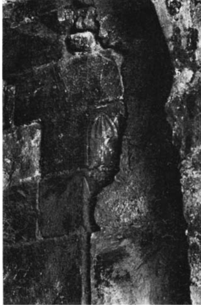
Plate 57.12 Muqarnaş springer in north wall of courtyard
