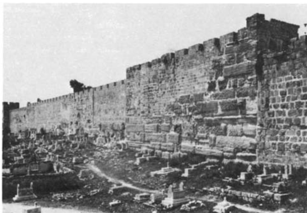
Plate 1 North-east corner of Ḥaram enclosing wall: east face
