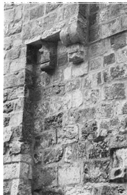
Plate 55.4 Roll corbels supporting extension of entrance salient
