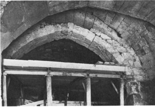
Plate 11.12 Vaulted bays of bridge across Tyropoeon Valley
