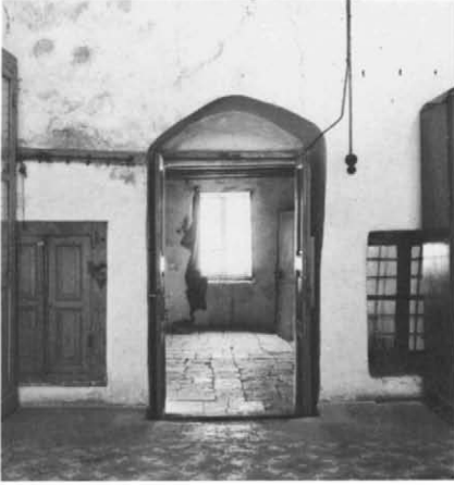
Plate 36.13 Upper floor: door and windows in rear wall of iwān
