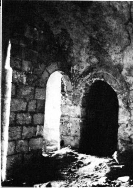
Plate 54.8 Door into room 'B' and entrance to staircase
