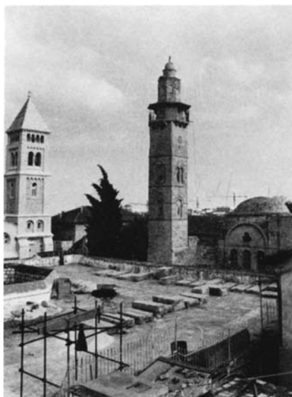
Plate 59.1 General view from north-west
