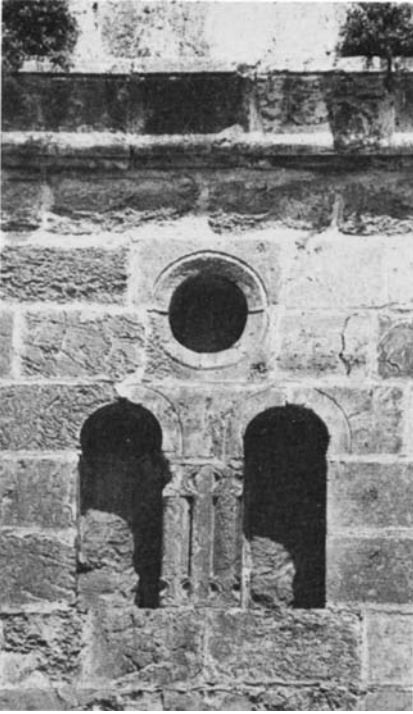
Plate 53.4 Blind triple window in façade
