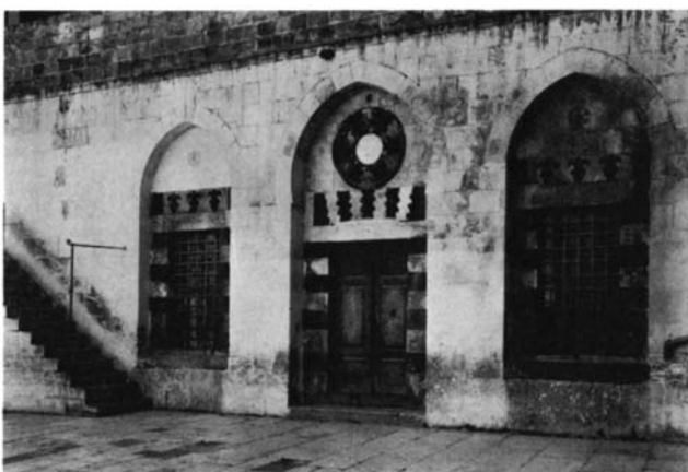
Plate 8.10 Façade of assembly hall to courtyard
