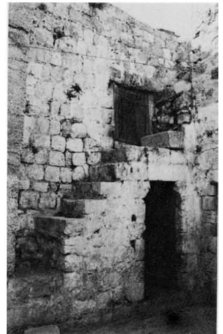
Plate 40.17 Upper floor: steps at west end of south wall
