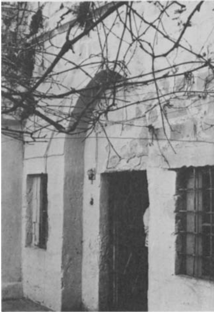
Plate 39.7 Doorway at east end of south side of courtyard
