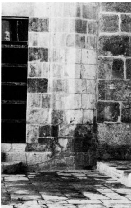
Plate 63.2 Top of half-arch at base of north wall of the assembly hall
