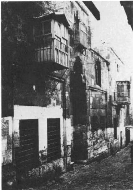
Plate 29.2 Façade from south-west
