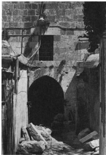
Plate 5.10 West face of doorway from vestibule to courtyard
