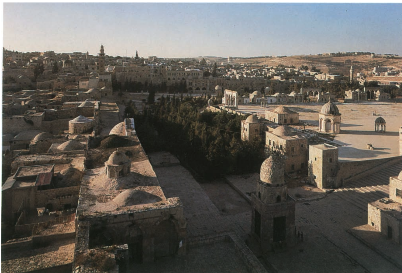
Plate 13 View north from Bāb al-Silsila Minaret
