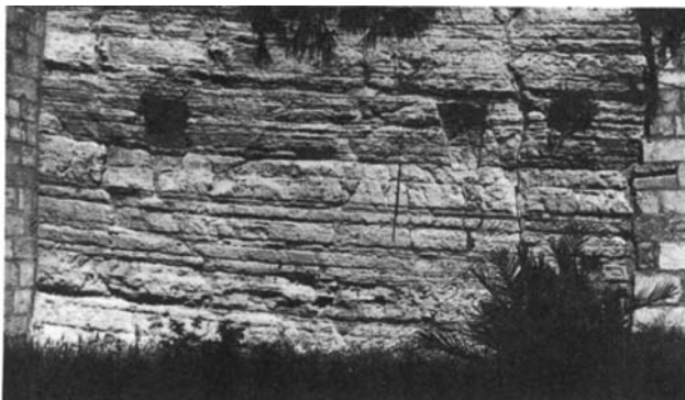
Plate 4 Empty sockets for vaulting springers in Antonia rock scarp
