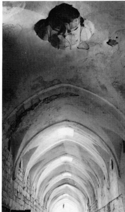
Plate 24.12 Vaulting, looking west, showing muqarnaş cupola at bay 17–18
