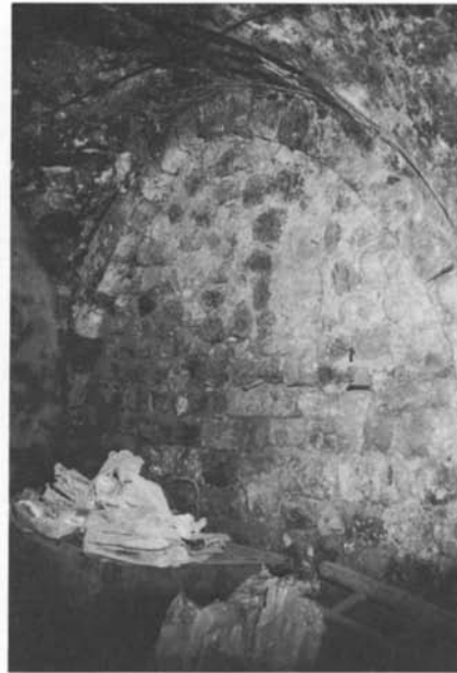
Plate 36.7 Blocked arch in west wall of hall 'C'
