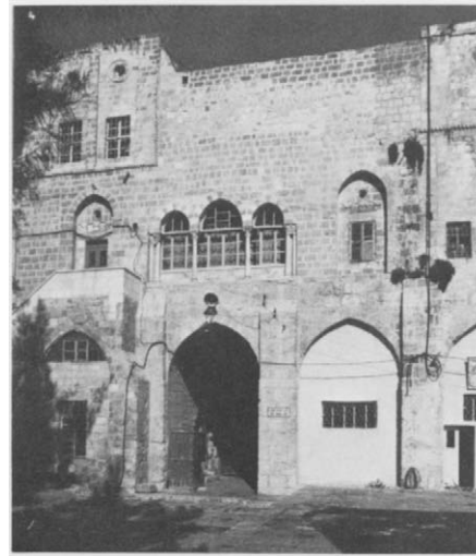
Plate 21.2 Amīniyya façade after restoration
