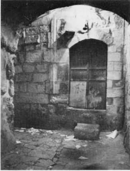
Plate 43.5 Window in south wall of tomb chamber seen from vestibule. (Lop-sided segmental arch, lowered sill and step are later alterations)
