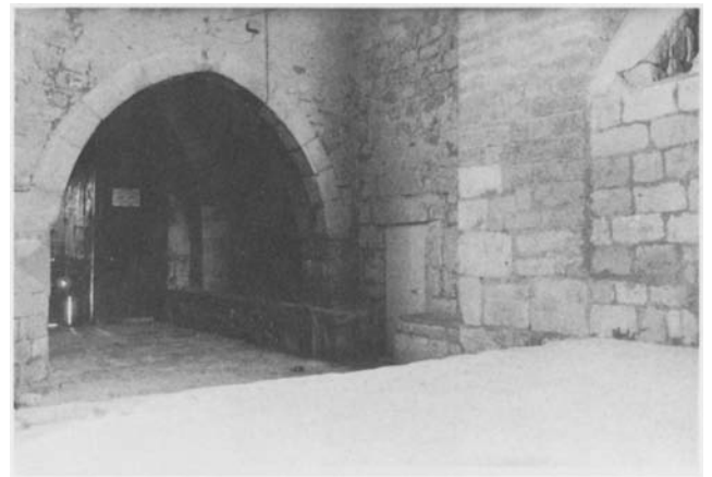
Plate 21.3 Street frontage, looking south-west
