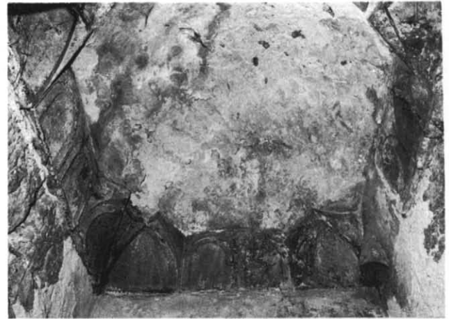
Plate 9.11 Remains of muqarnas corbelling in situ in room to east of corridor
