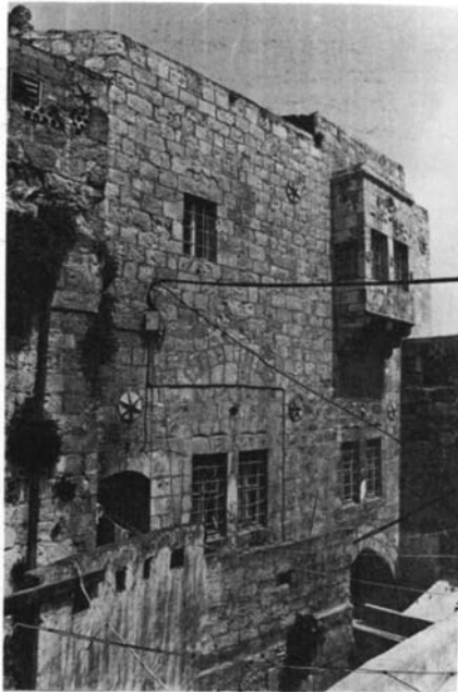
Plate 7.10 Three-storey Ottoman building to north
