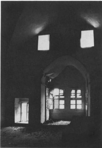
Plate 36.14 Upper floor: south end of main hall
