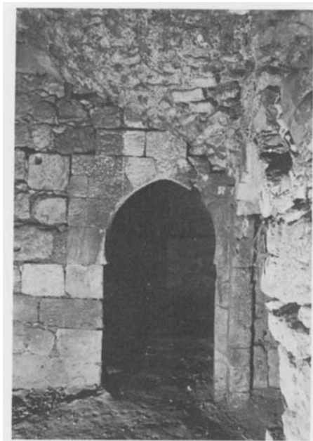
Plate 21.7 Mezzanine: door into south-western room 'A'
