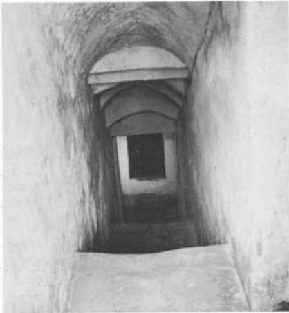
Plate 36.10 Looking down staircase towards mezzanine
