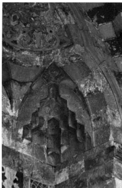
Plate 63.6 Squinch at right-hand (north) side of entrance portal
