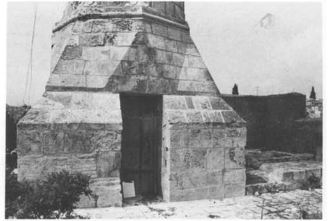
Plate 38.2 Entrance door in masonry plinth
