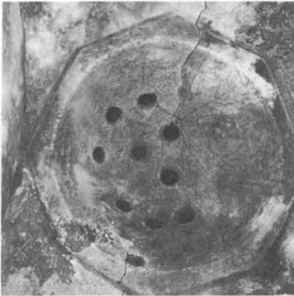
Plate 36.22 Upper floor: pierced dome of bath-house
