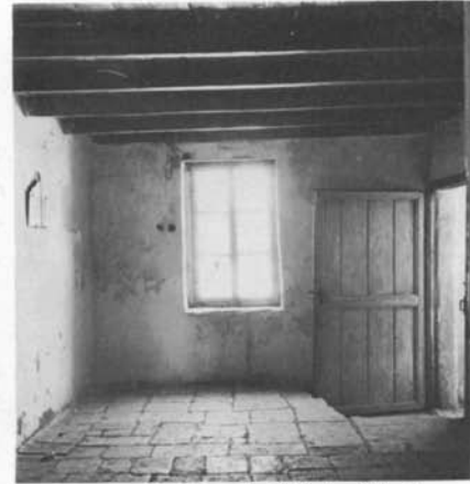
Plate 36.12 North end of (blocked) iwān showing beams supporting later floor
