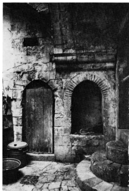
Plate 62.3 Arched well-recess with gadroon voussoirs and, above it, springing of later arch supporting extension to upper floor gallery
