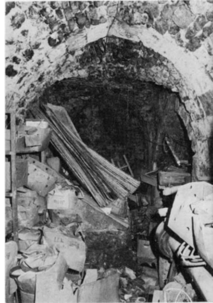
Plate 40.21 Southern vaults, looking west, with entrance from street vaults on right
