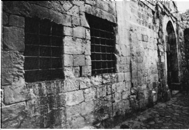
Plate 46.1 Street frontage from north showing tomb chamber windows
