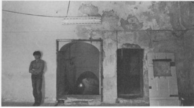
Plate 18.22 South wall of room 'J'
