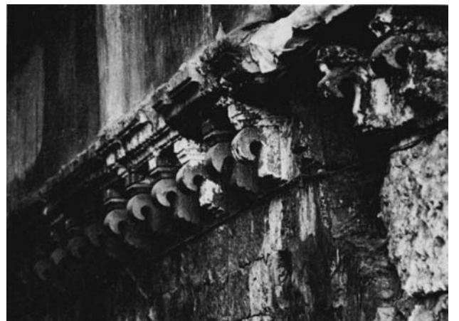
Plate 47.2 Details of corbelling
