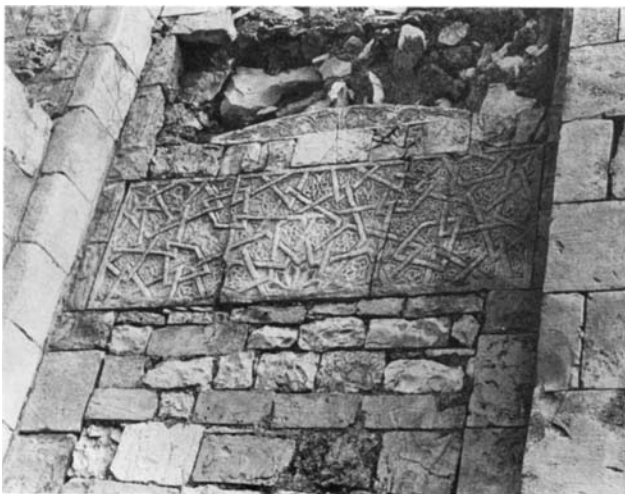
Plate 63.15 Lintel of window between outer court and west iwān
