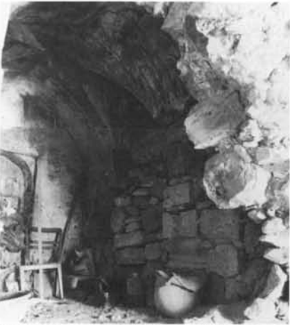
Plate 26.16 Upper floor: cell of Is'ardiyya through breach in west wall of Āmalikiyya cell
