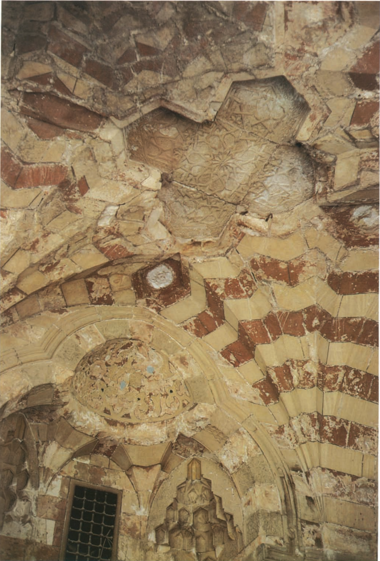
Plate 21 Vaulted ceiling above the entrance to the Ashrafiyya
