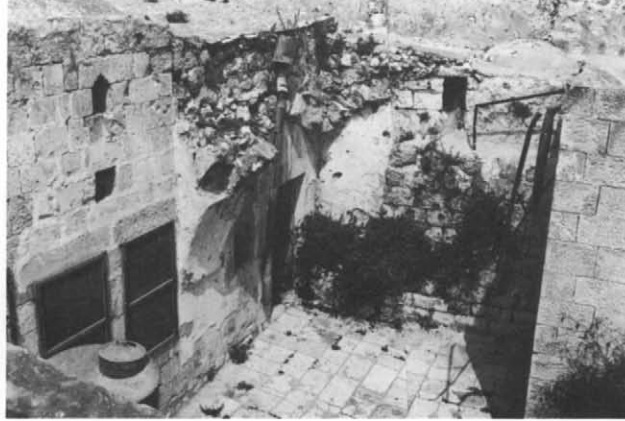
Plate 36.16 Upper floor: north-west corner of courtyard
