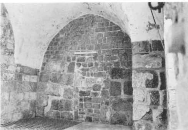
Plate 43.10 West wall of south iwān
