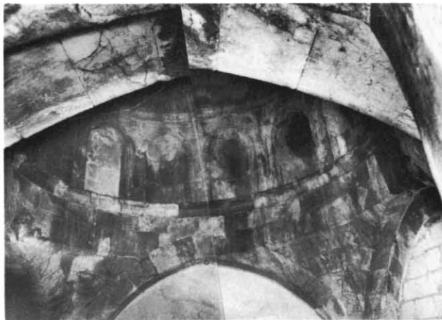
Plate 9.9 Tomb chamber: zone of transition
