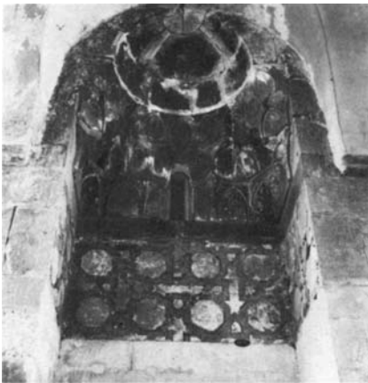
Plate 13.3 Head of entrance portal
