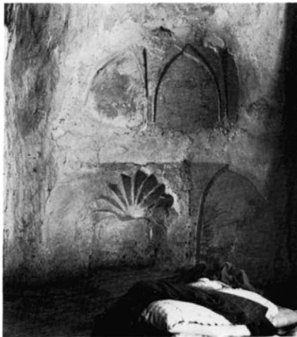
Plate 24.11 Muqarnaş fragments in room above bays 29–30
