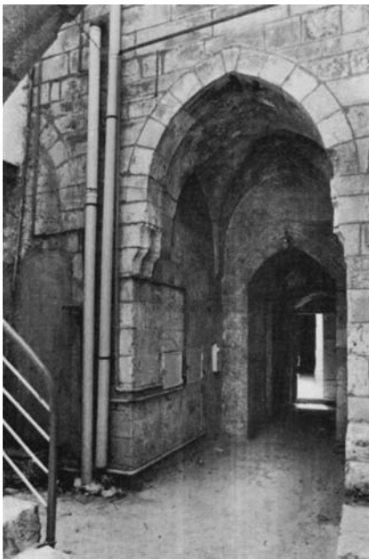
Plate 58.5 Vaults at south end of courtyard
