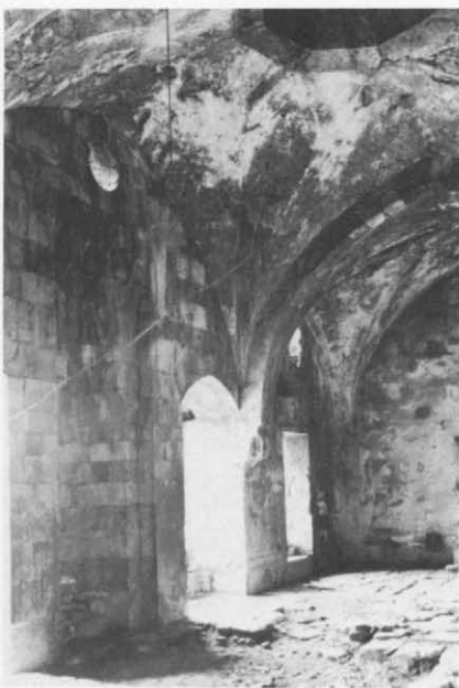
Plate 33.5 South wall of assembly hall
