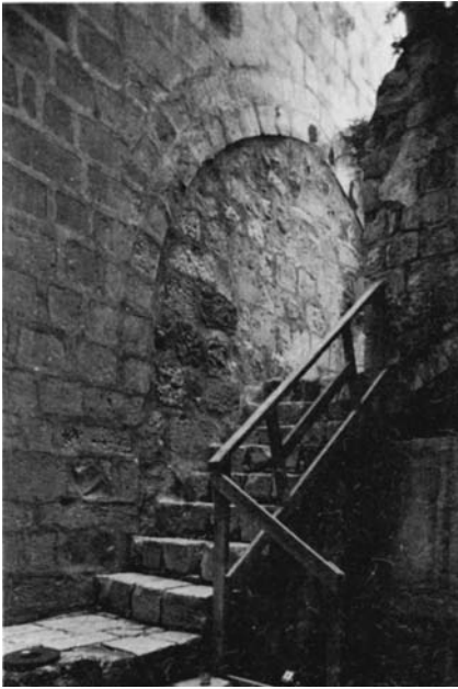
Plate 57.11 Blocked archway in the south wall of the courtyard
