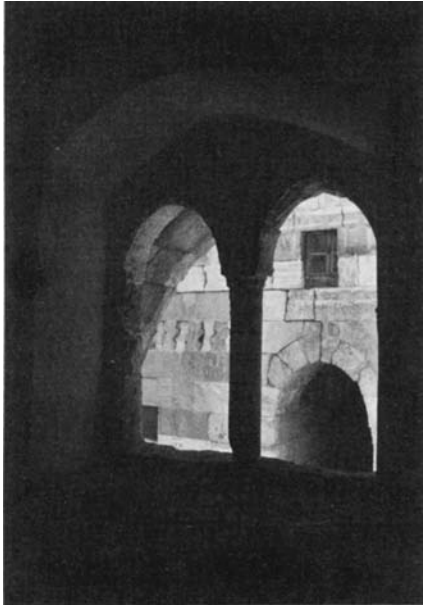
Plate 58.10 Window of mezzanine overlooking street
