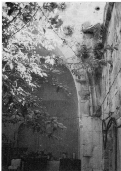
Plate 42.7 West abutment of iwān arch
