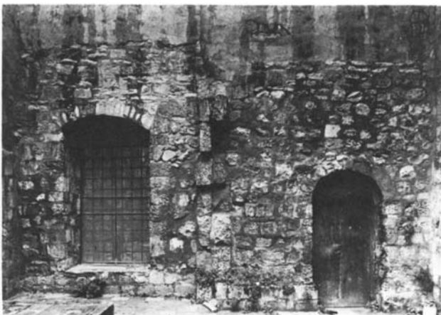
Plate 2.2 North side of courtyard
