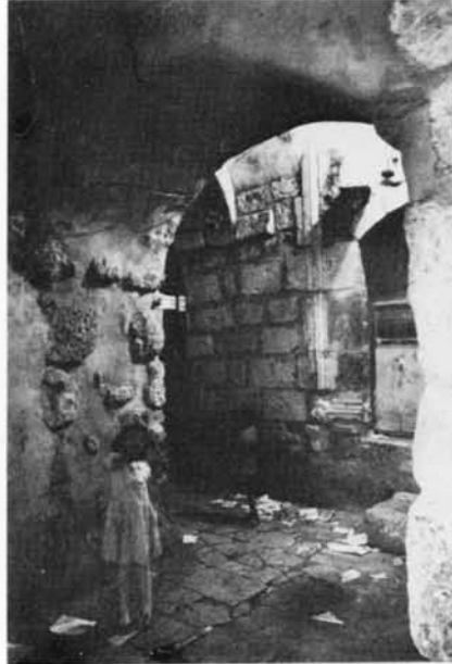
Plate 43.6 South end of entrance corridor
