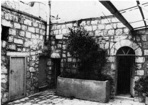
Plate 55.7 North-west corner of courtyard
