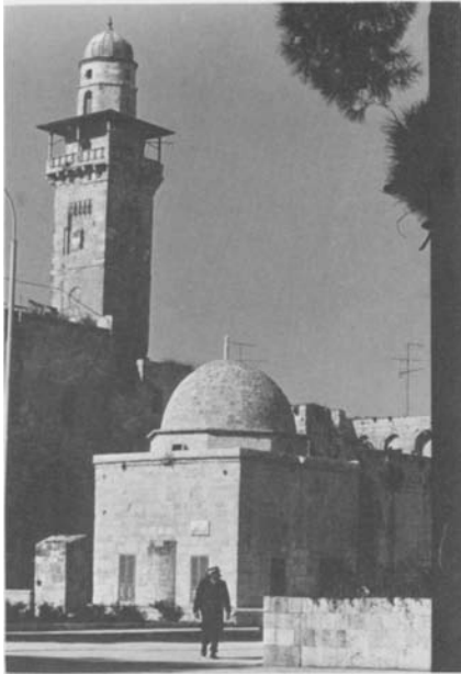
Plate 20.1 General view from south-east with Qubbat Mūsā (647/1249-50) in foreground
