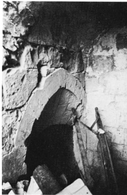
Plate 48.12 East side of doorway from west vestibule to main staircase
