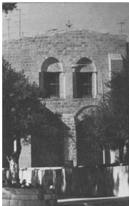
Plate 18.3 Central windows after repairs made in 1979
