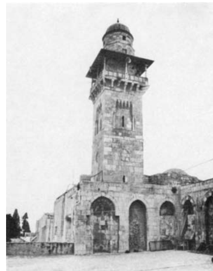
Plate 63.19 Remains of south wall of madrasa, showing mihṛāb and Bāb al-Silsila Minaret
