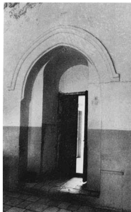
Plate 53.7 Doorway in north wall of room 'B'
