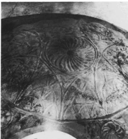
Plate 36.18 Upper floor: domical vault
