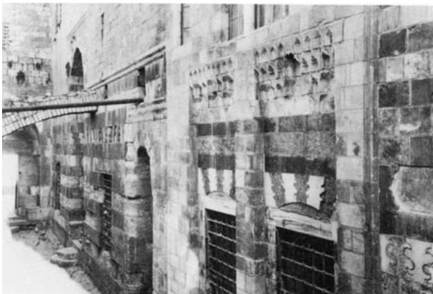
Plate 62.2 Paired windows in façade, with Arghūniyya beyond
