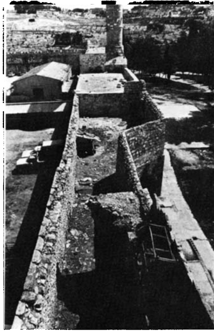
Plate 54.10 Roof of Ghādiriyya, from the west
