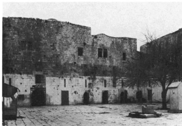
Plate 5.8 East side of courtyard
