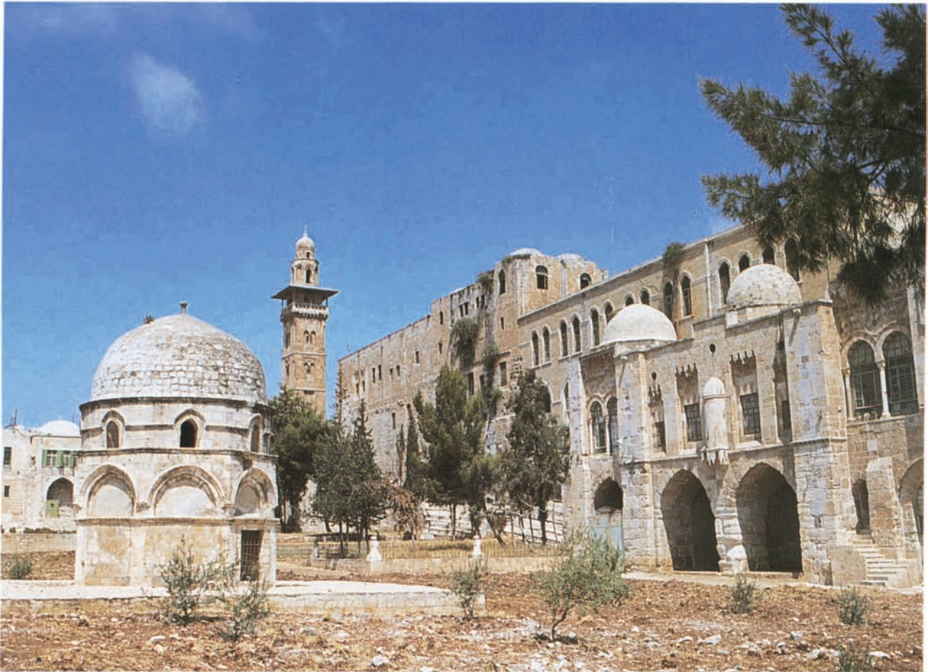
Plate 22 Left, Qubbat Sulaymān; and the north side of the Haram
