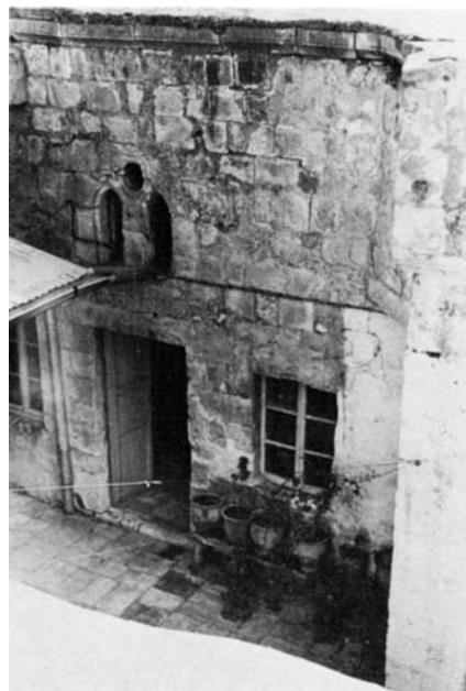
Plate 55.8 Entrance to assembly hall
