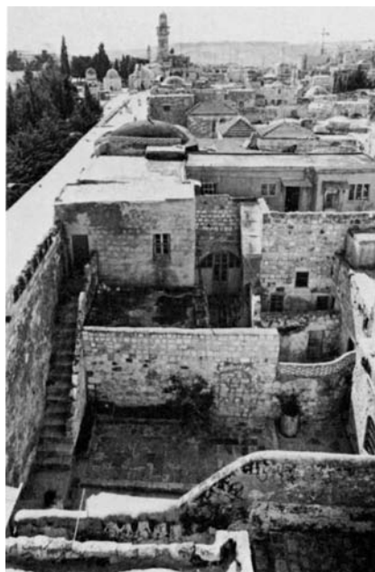
Plate 44.2 General view of upper floor, looking south
