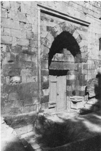
Plate 54.2 Entrance portal with excavated pavement in foreground
