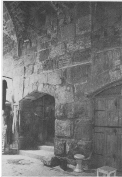
Plate 24.1 Masonry joint between bays 16 and 17 (north side)
