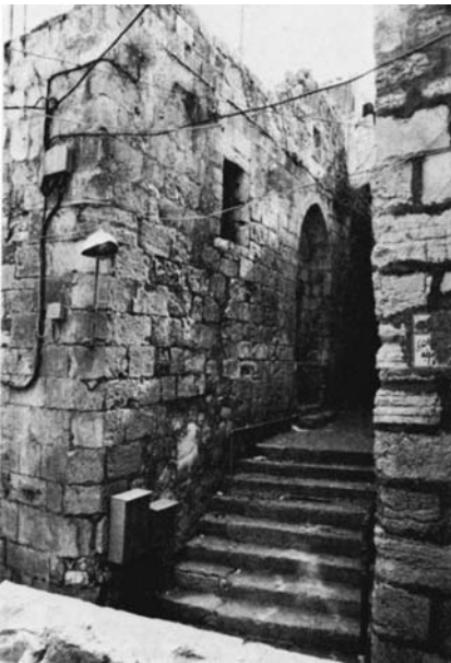
Plate 48.7 Entrance in west frontage of western annex
