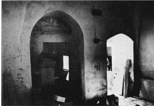
Plate 48.18 Upper floor: east wall of room at north-west corner of courtyard
