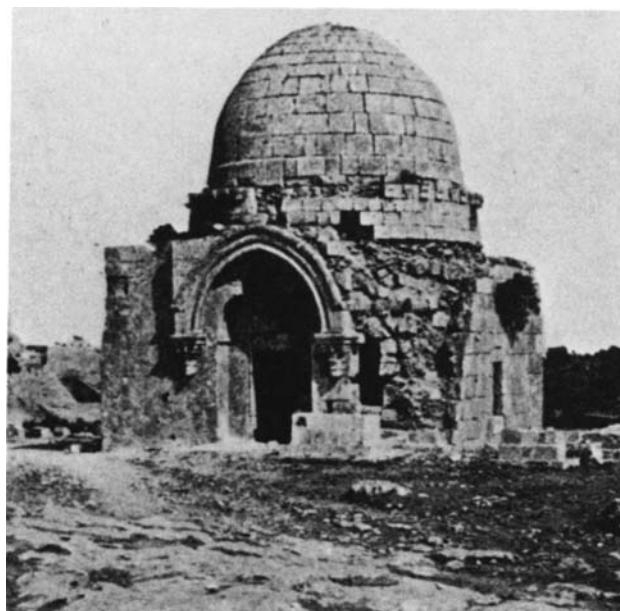
Plate 6.2 Dilapidated state of building in 1877 (After a photograph by Felix Bonfils)
