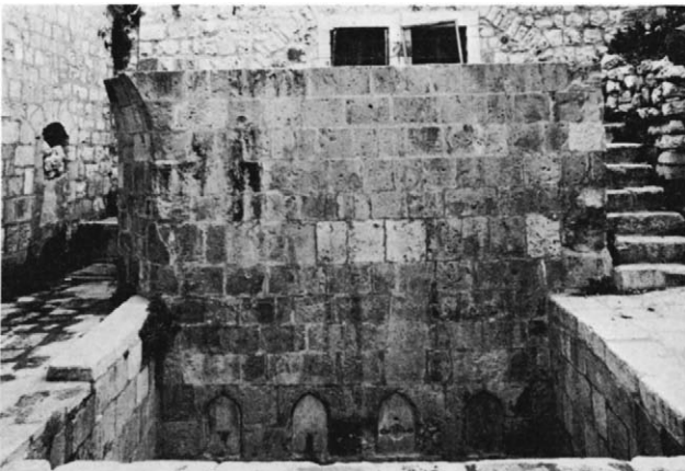
Plate 48.19 Water fountain in east yard
