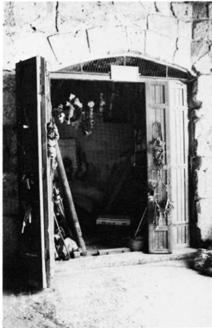
Plate 24.24 Shop on south side, bay 1
