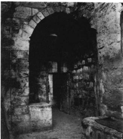
Plate 3.12 Entrance door from the interior, looking south
