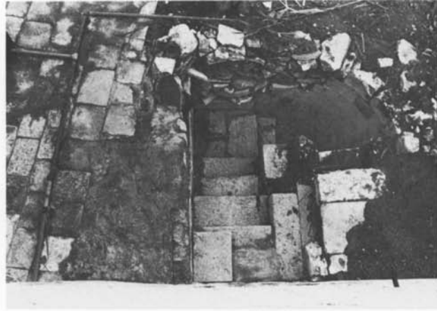
Plate 33.26 Staircase emerging at upper floor level
