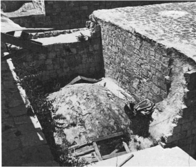
Plate 11.2 Dome surrounded by later structures
