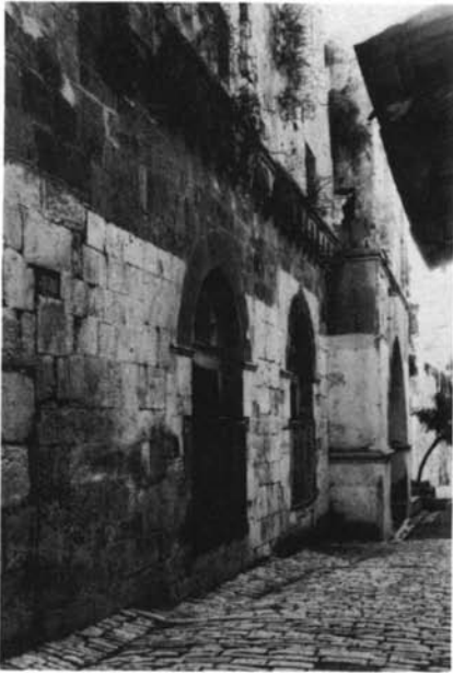
Plate 5.1 Eastern end of street façade
