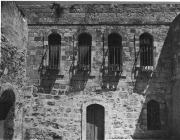
Plate 2.8 East side of courtyard
