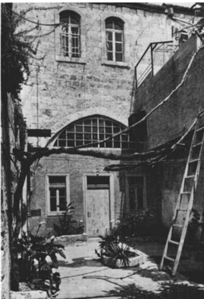
Plate 58.7 Ṭwān at north end of courtyard (with modern structure above)
