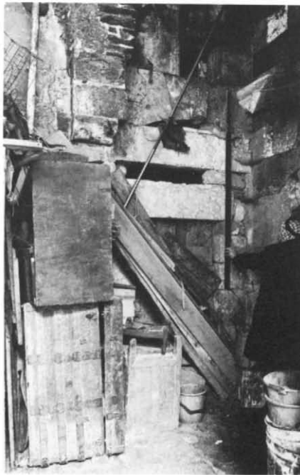
Plate 25.11 Door into corridor at north-east corner of courtyard
