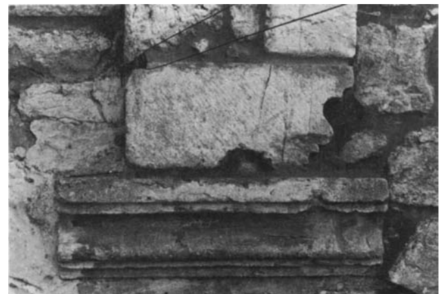
Plate 15.4 Re-used mouldings at south-west corner of landing
