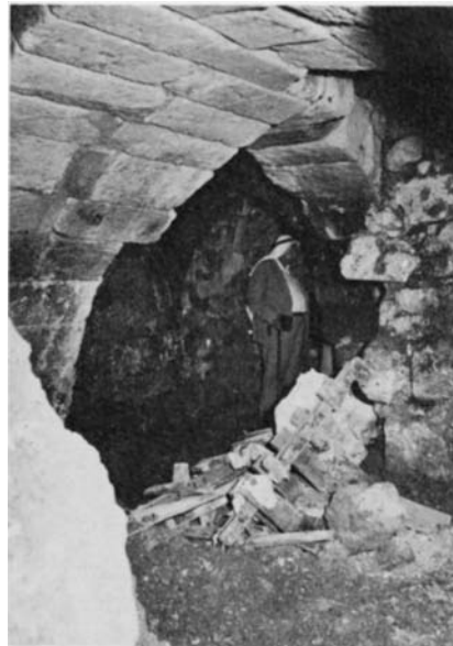
Plate 40.12 Earlier structures in south-west corner
