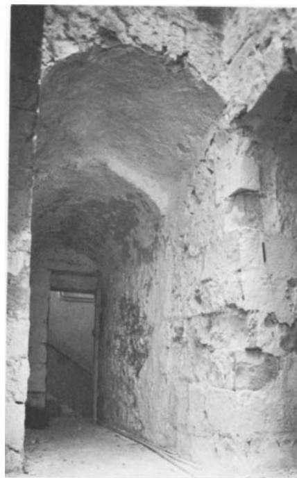
Plate 18.19 Mezzanine corridor, looking south
