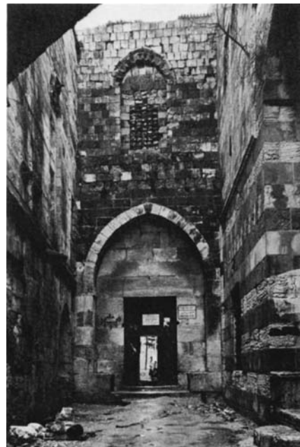
Plate 58.13 Bāb al-Hadīd, showing window of assembly hall above
