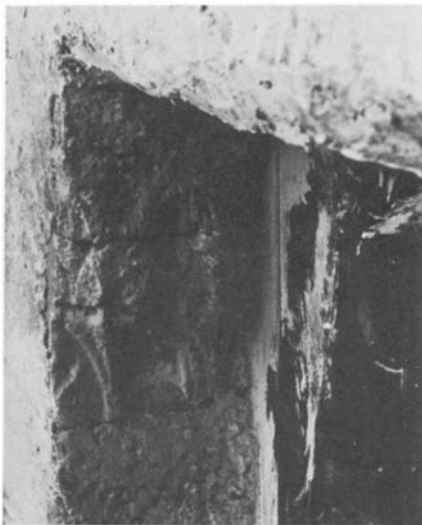
Plate 39.5 Muqarnas shoulder at left-hand side of entrance door
