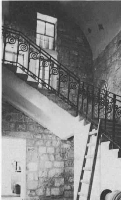
Plate 35.19 Stairwell, looking west
