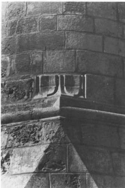
Plate 38.3 Detail of transition from base to shaft
