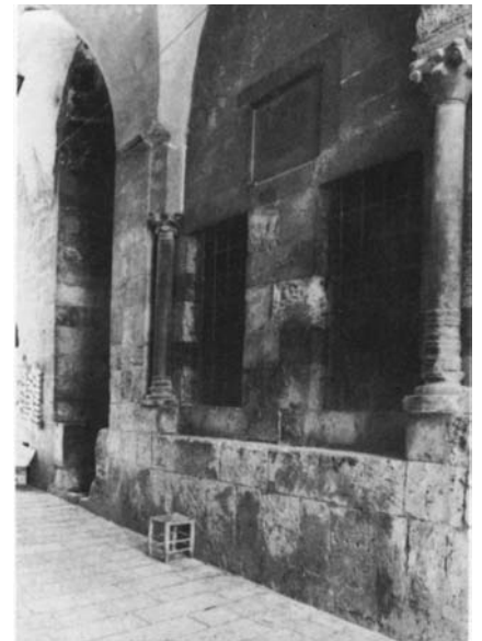
Plate 13.1 Street façade from south-east
