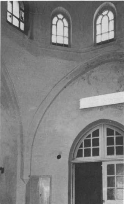
Plate 35.18 South-west corner of loggia
