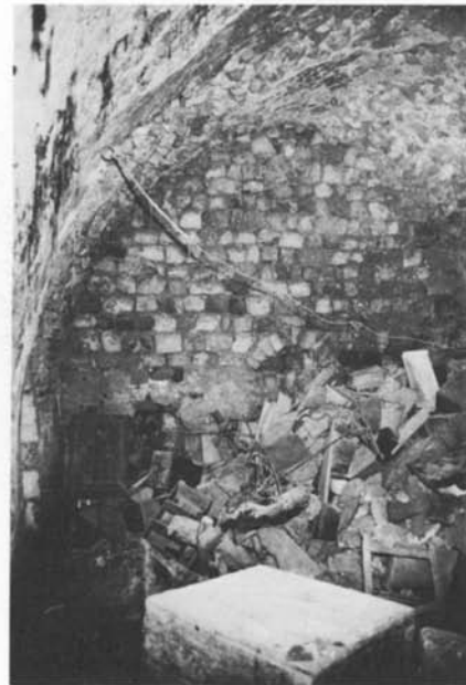
Plate 36.9 West end of hall 'D'
