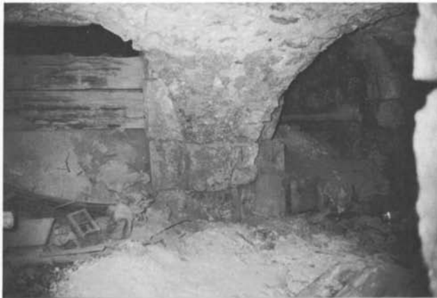
Plate 36.8 Openings in west wall of hall 'C'
