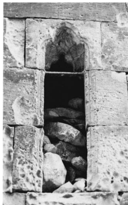
Plate 49.3 Slit window at west end of street façade
