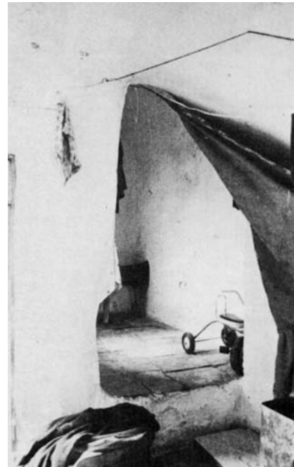
Plate 43.24 South-east mezzanine: ancillary chamber to north
