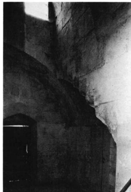
Plate 8.12 Lobby at north-east corner of courtyard: north-east corner
