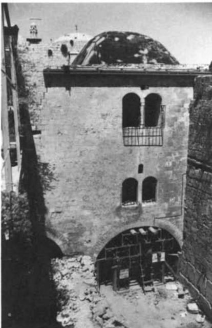
Plate 7.6 Modern structures at north end of courtyard
