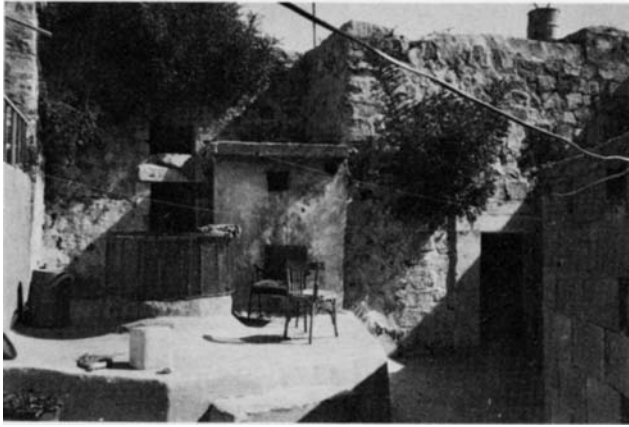
Plate 40.14 Upper floor: general view to east
