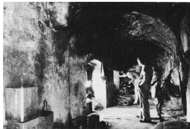
Plate 62.8 Upper floor room ' K^2 ' looking east
