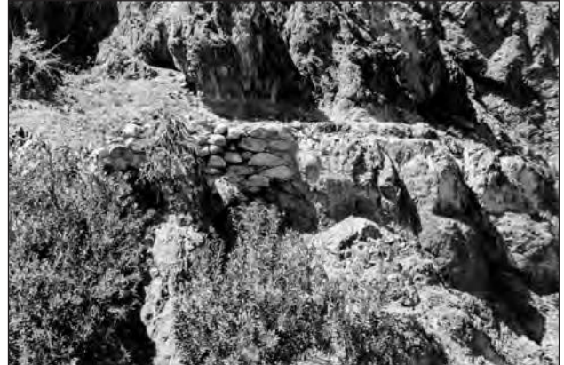
Figure 5.39 The rock-cut aqueduct conduits feeding water from the Wadi Ghuwayr springs to the large reservoir and mill (WF11) complex. There are traces of two or three phases of remodelling, marked by different channel recuts in the rock wall at different levels. (Photograph: Darren Crook.)
