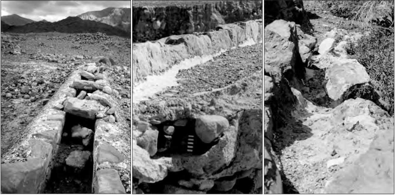
Figure 4.33 Three sections of the channel of aqueduct WF31/WF33: (left) the well-preserved extension to the aqueduct feeding the mill at WF11, looking east; (centre) detail of channel on aqueduct bridge over Wadi Shayqar, showing two phases of waterproof lining (lower marked by 10 cm scale), looking west; (right) rock-cut channel in south edge of Wadi Ghuwayr gorge, looking west. Scale: 1 m. (Photographs: Darren Crook.)
