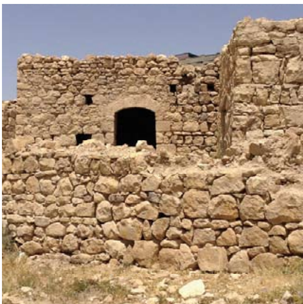
Figure 11 Old houses in Basta
