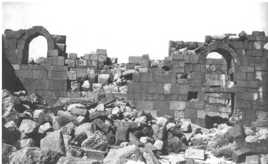
Fig. 10.7: Qasr el-Hallabat : Crawford's view of the courtyard wall of Rooms 10 and 11 in 1928 when they still stood two storeys high. Note the building inscription of 529 in place below the window on the left. The Latin inscription of 212–214 was apparently also once set in this wall.
