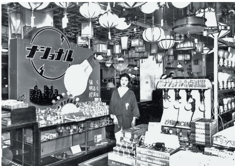
5.9 Matsushita National brand store interior, display with sample bulbs and slogan “strong, bright, economical,” ca. 1930s. Panasonic Operational Excellence Co., Ltd.
