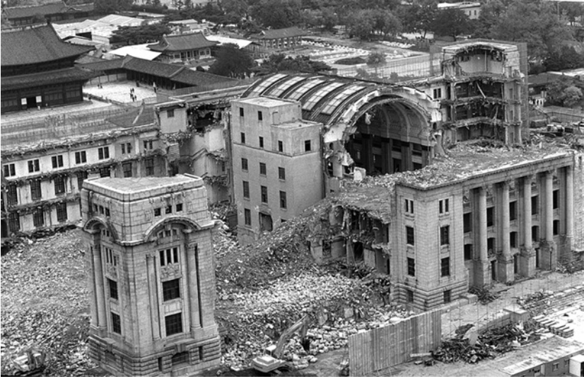
FIGURE 3.1. Demolition of the former Japanese governor-general building, Seoul, 1996.
