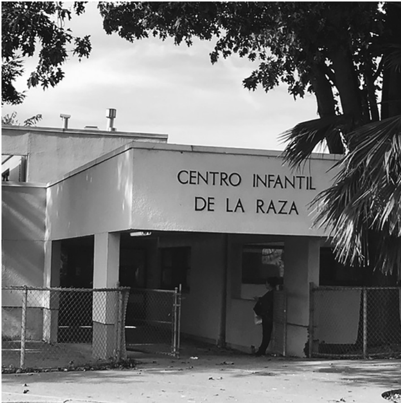
1.7 Offices of Centro Infantil. The school remains in the same location, but new additions have been built. Photograph by Annette Oropeza.
