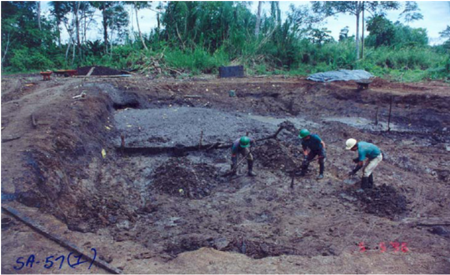
FIGURE 29 Oil well Sacha-57 (pit #1) during Texaco's remedial action plan (RAP). Taken by Woodward-Clyde (the environmental remediation contractor) on May 5, 1996, the photo depicts heavy crude embedded at the bottom of the pit after liquids and viscous hydrocarbon contents were removed. Source: Maria Aguinda Salazar y Otros v. ChevronTexaco Corp. , Case No. 002-2003-P-CSJNL (2011-63-1), p. 11,849, Provincial Court of Justice of Sucumbíos, Nueva Loja, Ecuador.
