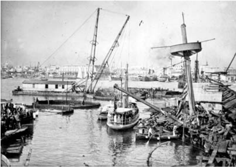
Figure 1.5 Maine in cofferdam, Havana. Source: Library of Congress. Prints and Photographs Division.
