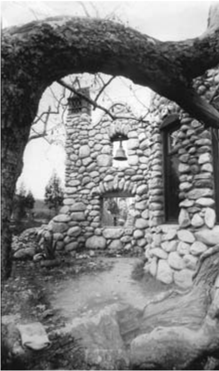
Exterior view of the Charles Fletcher Lummis home, El Alisal, under construction, Los Angeles, 1890s.
