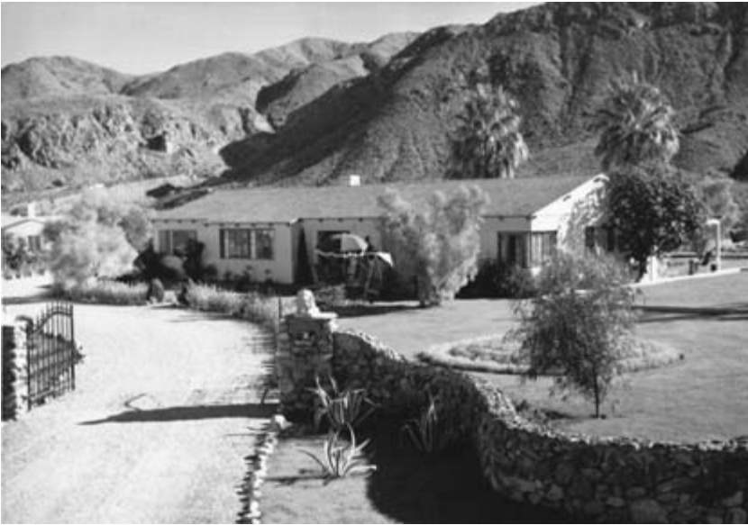
Dick Richards home, Smoke Tree Ranch, Palm Springs, California, 1930s. Photograph copyright held by Palm Springs Historical Society, Palm Springs, California, courtesy Palm Springs Historical Society, Palm Springs, California.
