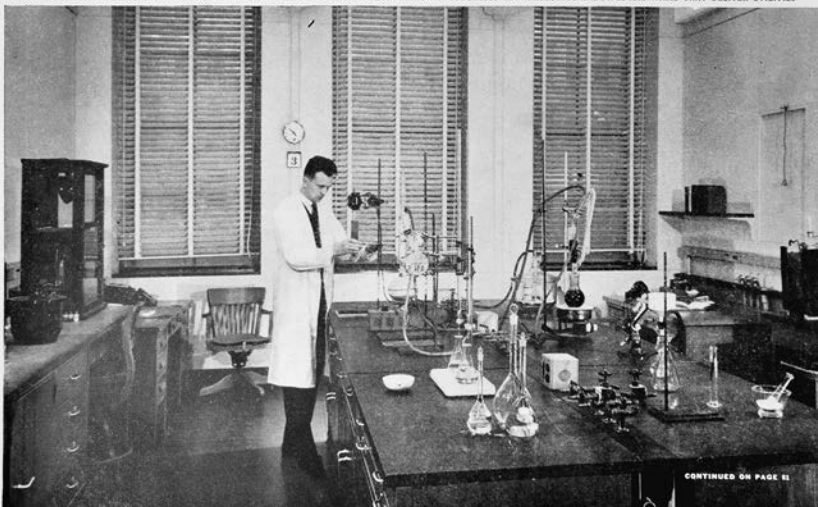
WITHIN 48 HOURS COMPLETED LABORATORY IS AT WORK. WALL HAS BEEN INSTALLED AT RIGHT. CONCEALED IN WAINSCOTING ARE PIPES AND WIRES THAT DELIVER UTILITIES
