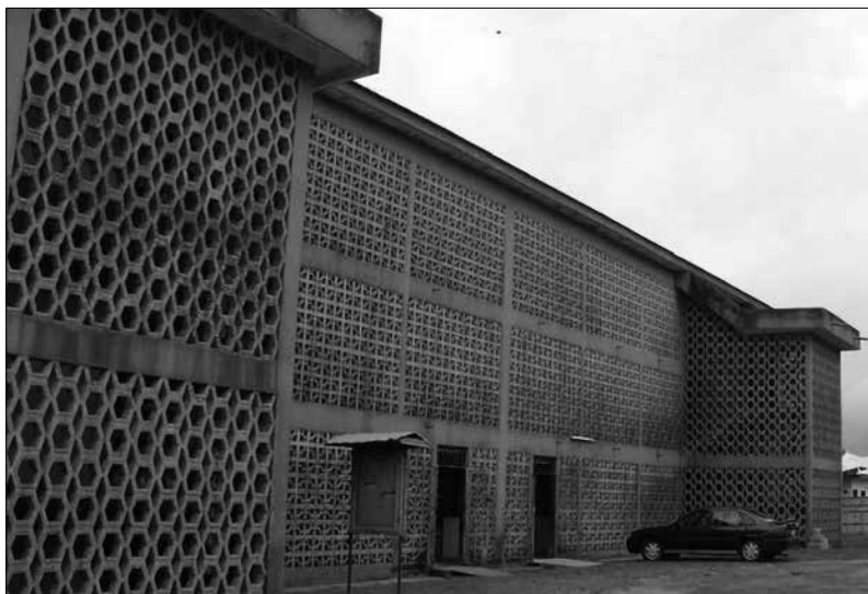
FIGURE 5.4. Multistory building with walled-off exterior. Author photo.
