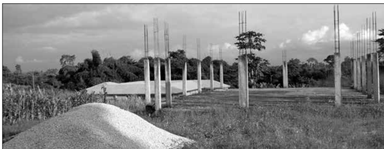
FIGURE 5.1. Unfinished assembly building five years into construction, Eastern Region. Author photo.
