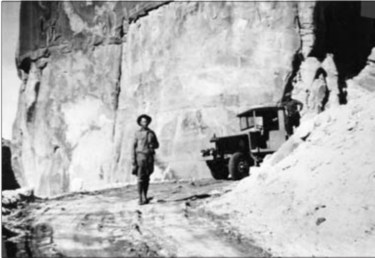
Working on the entrance road to Horseshoe Canyon, 1929. Lou Chaffin in road, Clell Chaffin on the truck bed. Photo courtesy of Ned Chaffin.
