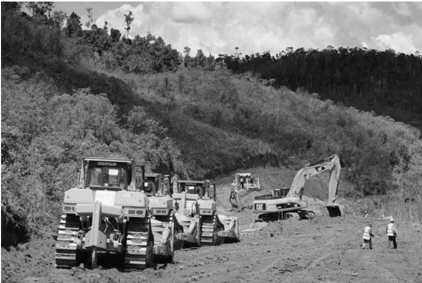
Figure 10 Earth movers used to clear swaths of primary and secondary forests to build the 220 km-long pipeline in 2008. (Photo by Roberto Schmidt/AFP via Getty Images)
