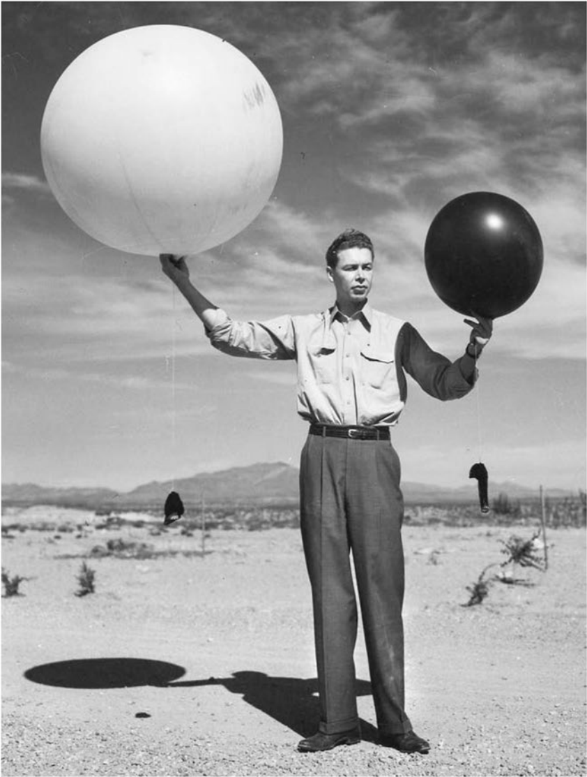
FIGURE 2.5. Weather balloons carrying mesh bags filled with dry ice during artificial nucleation experiments in New Mexico. From C. R. Holmes and William Hume II, "Final Research Report to the State of New Mexico Economic Development Commission Water Resources Development," New Mexico Institute of Mining and Technology, September 1951.
